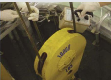
Preparing HEU for removal from a research reactor core to allow for conversion to LEU
